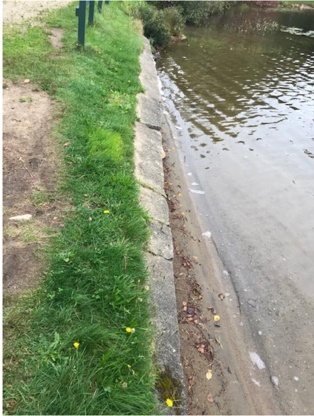
Existing northern retaining wall
