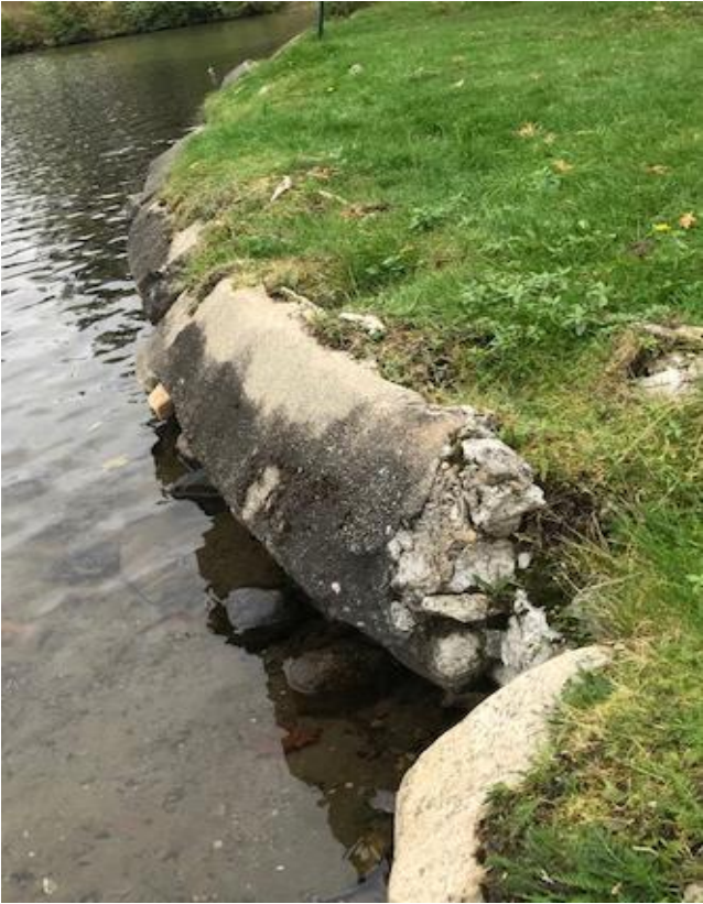
Existing southern retaining wall
